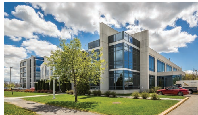
Intrado Life & Safety Canada Inc. 7150 Alexander-Fleming Street, Saint-Laurent, QC
