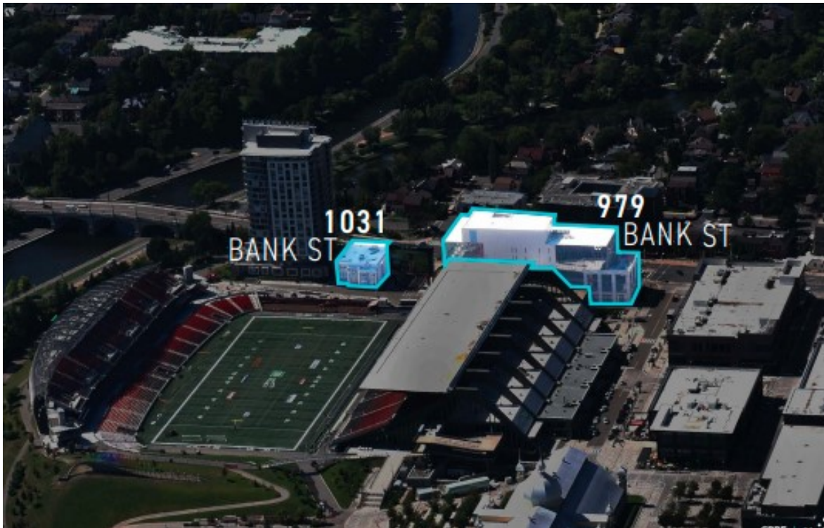
Aerial view of 979-1031 Bank Street
