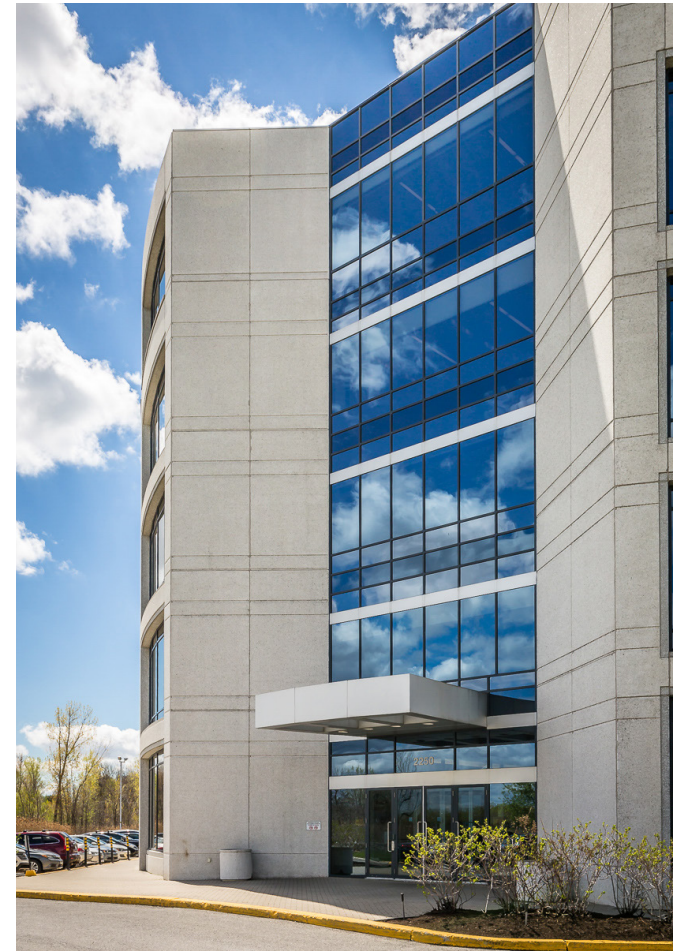
LED lighting retrofit in 2022 2250 Alfred-Nobel Boulevard, St-Laurent, QC
