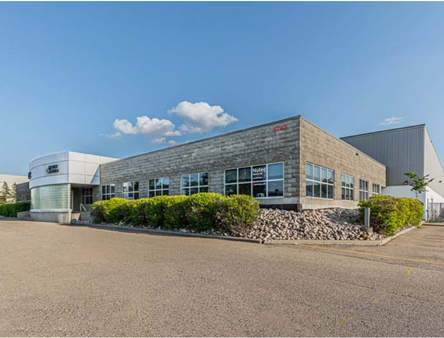
8743 50 th Avenue NW, Edmonton, AB
