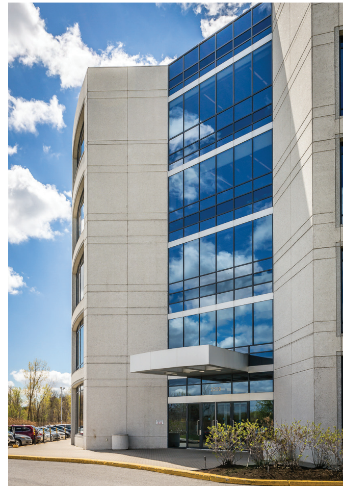
LED lighting retrofit in 2022 2250 Alfred-Nobel, St-Laurent, QC
