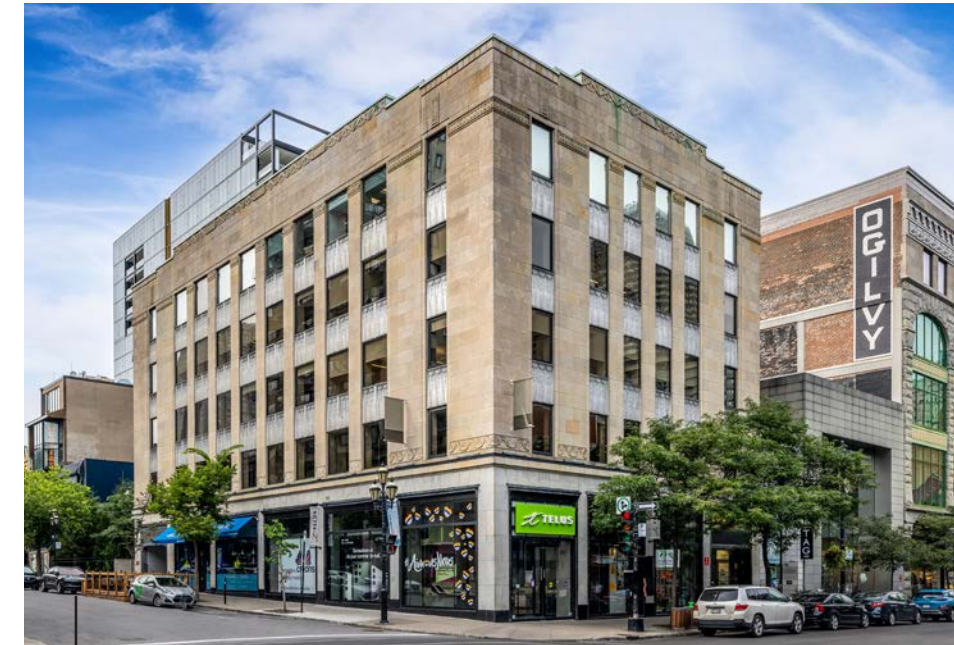
1327-1333 Sainte-Catherine Street West & 1407-1411 Crescent Street, Montréal, QC
